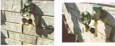
Picture of typical hose connector. Small. When tightened to hose bib, diverter handles often face the wall. Notice in the side view in figure 2, valve handle sticks out further than the diverters—making it difficult to hook up hose or to turn the diverters (in technical talk—a knuckle buster).
